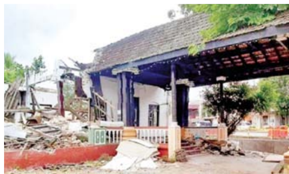
The demolished Bhuwenekabahu Hotel.
