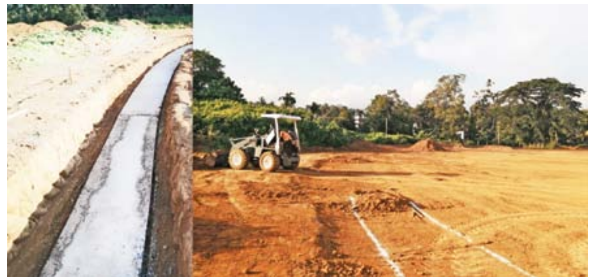
Construction work continues at the Ratnapura ground.
