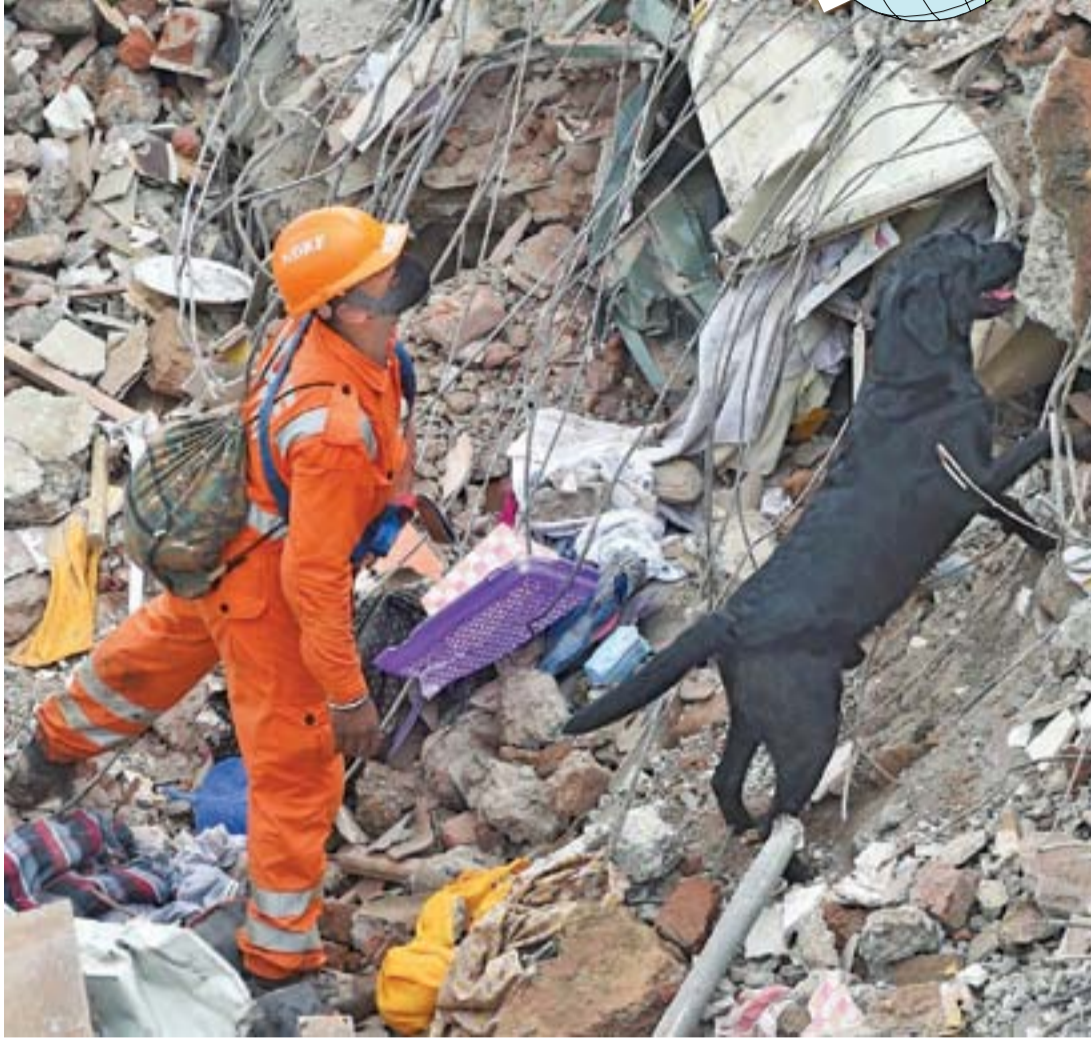
A rescue worker along with a sniffer dog searches for survivors in the rubble of a collapsed five-storey apartment building in Mahad, India on Tuesday. - AFP
