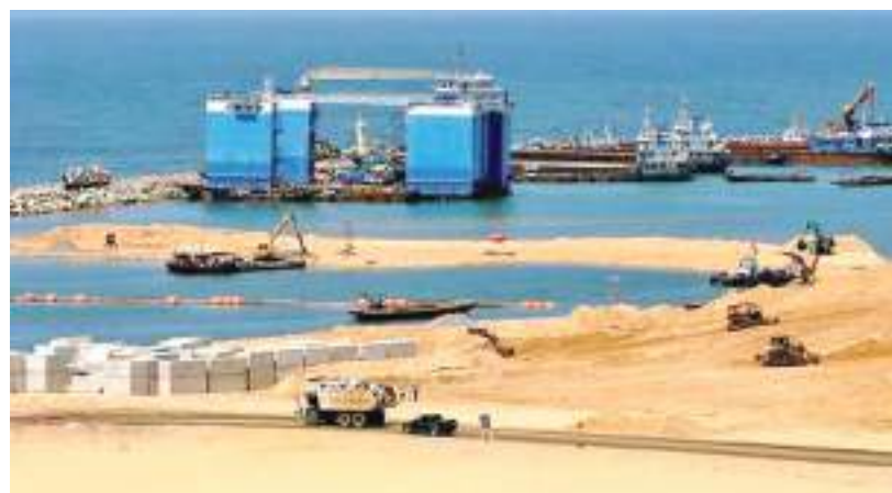
The East Container Terminal Project.
