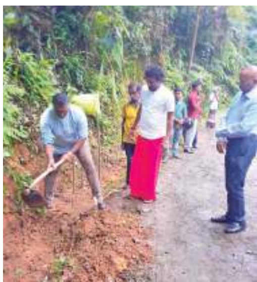
The road rehabilitation work in progress.
