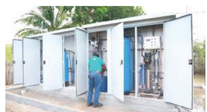
The water purification plant
