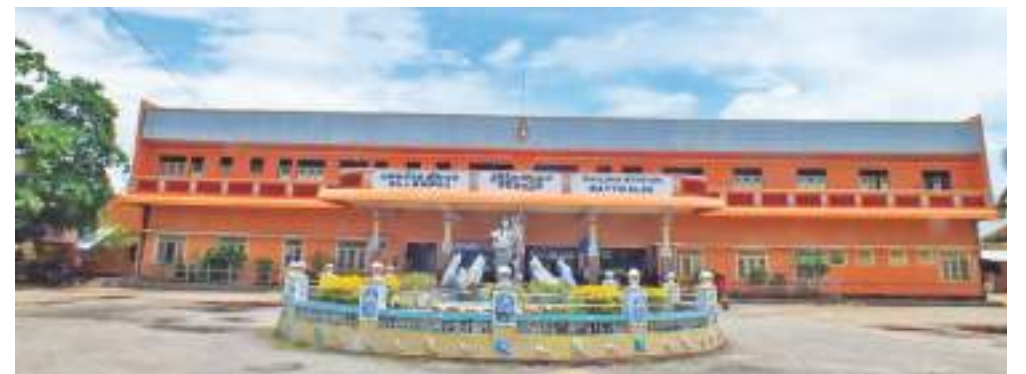
The Batticaloa Railway Station.
