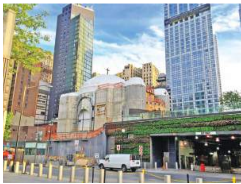
St. Nicholas Greek Orthodox Church being rebuilt.
