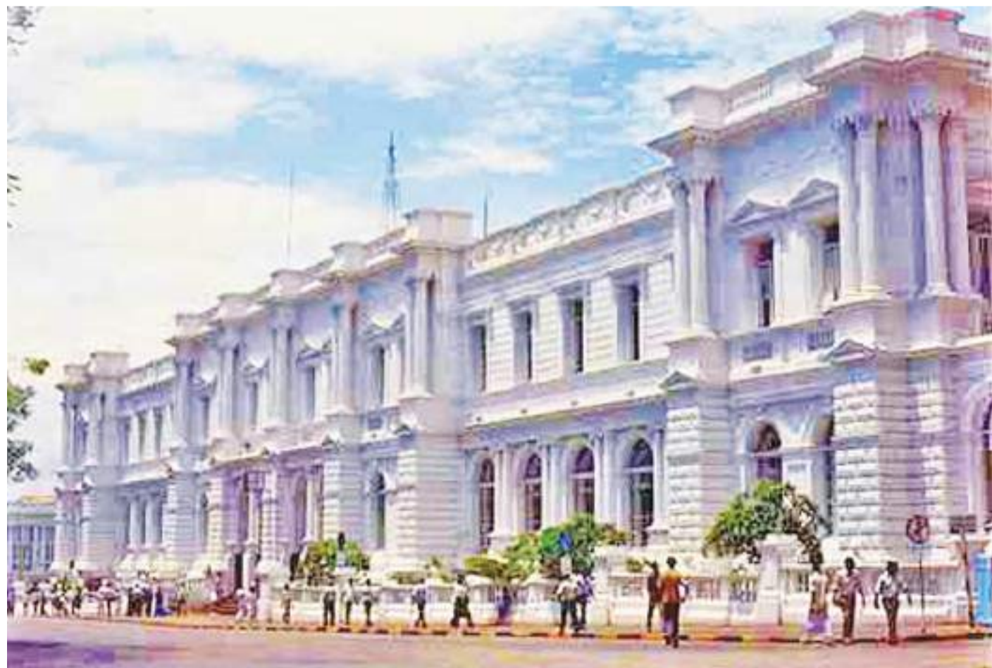
The old General Post Office, Colombo
