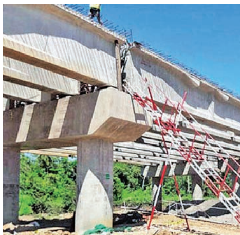
The Central Expressway under construction.
