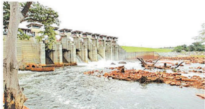
The Deduru Oya Reservoir
