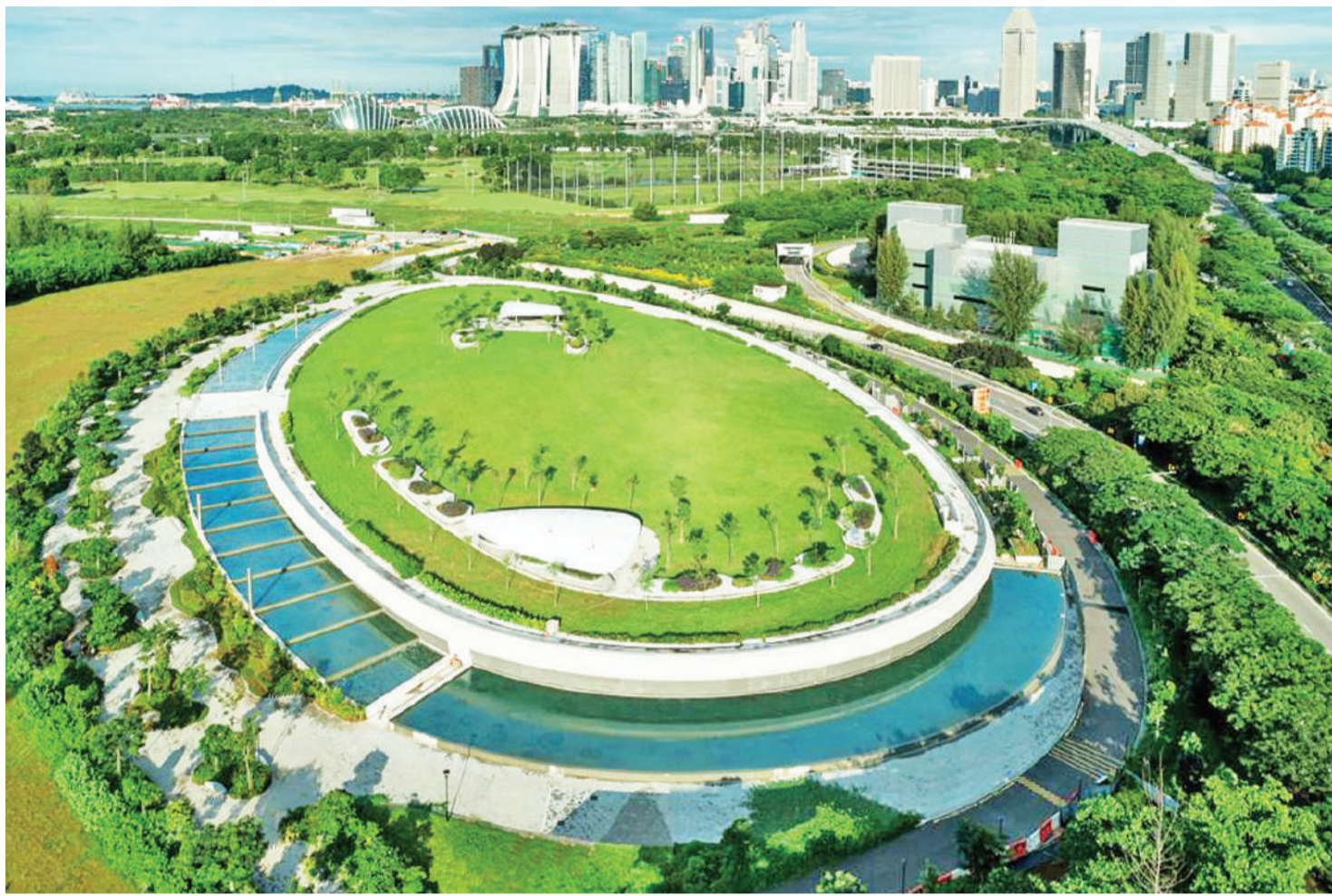
The Keppel Marina East Desalination Plant. Governments need to work closely with the private sector to accelerate the green transition. While governments can set the direction with policies, industry players hold the expertise to introduce innovative green solutions.
