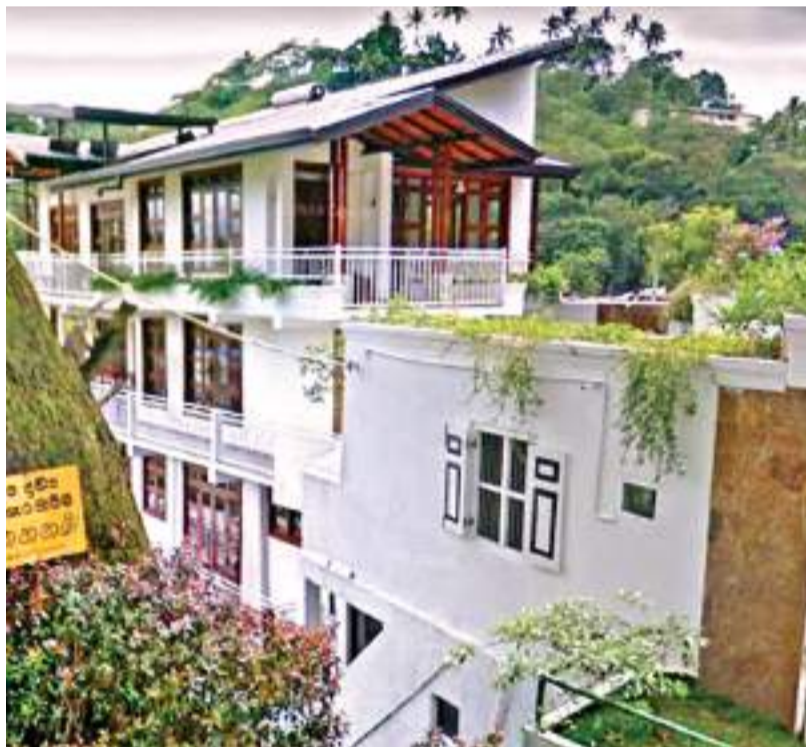
The house before collapse
