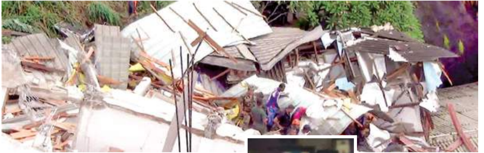
The house after collapse
