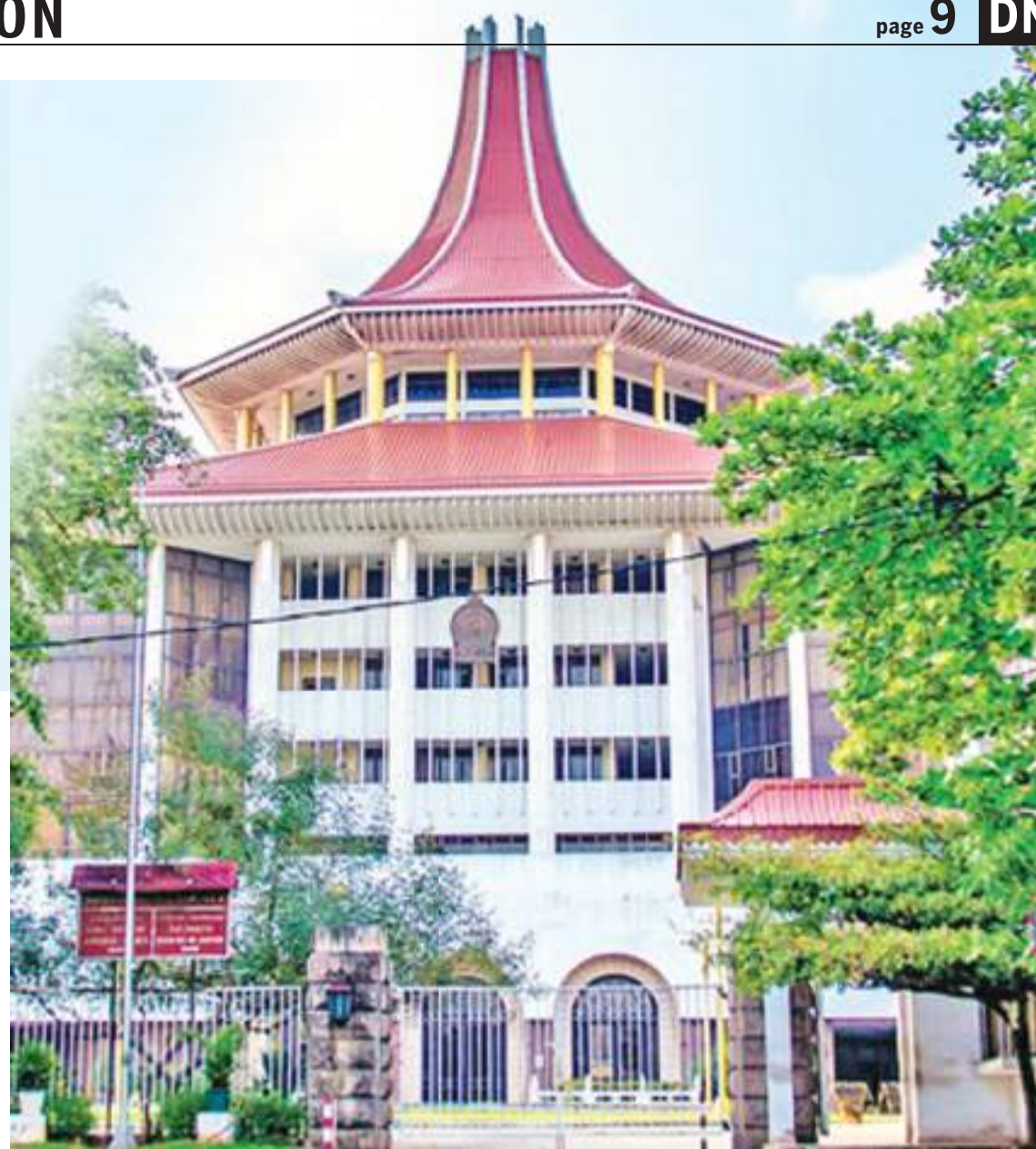
The Supreme Court Complex in Hulftsdorp, Colombo 12.
