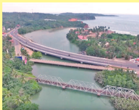
Polwathumodara Bridge in the Southern Province.
