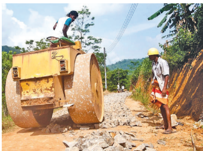
The Government is repairing 100,000 Km of rural roads
