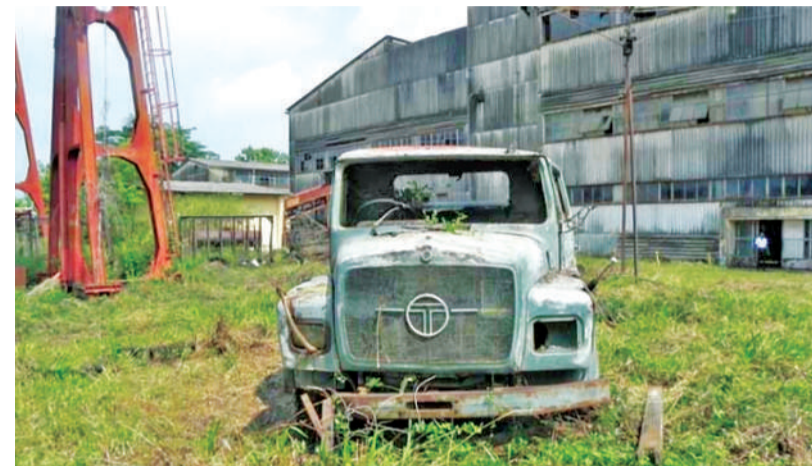
The Kantale Sugar Factory which was written off and left to ruin
