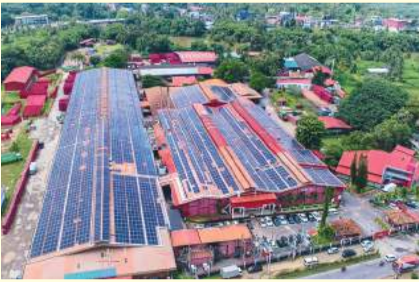
One of the largest single location rooftop solar projects in Sri Lanka at the Coca-Cola Beverages Sri Lanka Ltd. plant in Biyagama
