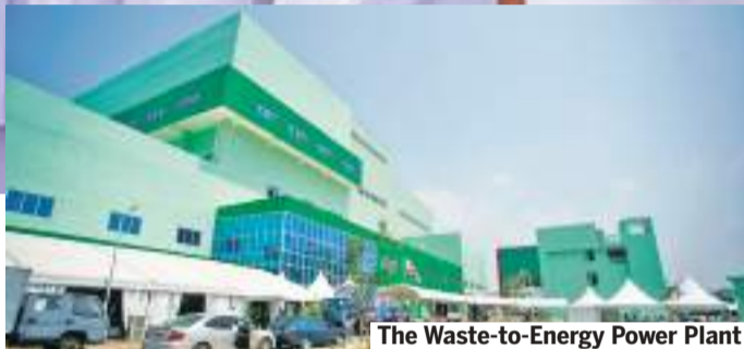
The Waste-to-Energy Power Plant
