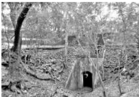
Tunnel on Sober Island
