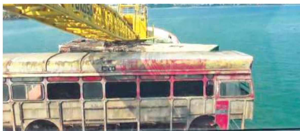
A discarded bus being lifted to be submerged.
