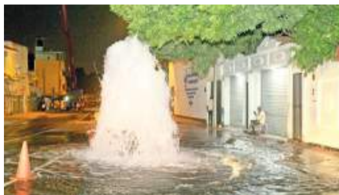
A burst pipeline at Siri Dhamma Mawatha, Colombo 10 was left unattended for several hours on Wednesday night, causing a mini-flood in the area. Picture by Sulochana Gamage
