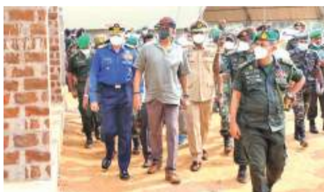
Defence Secretary Gen. (Rtd.) Kamal Gunaratne and other officials inspecting one of the construction sites. Picture by Rukmal Gamage.
