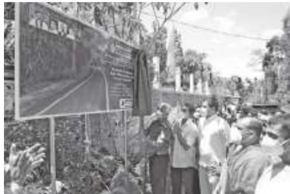
Inaugurating the road work.
