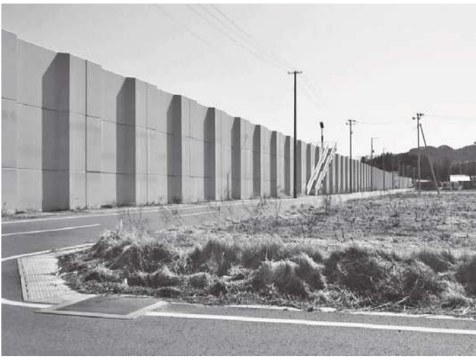
Twelve and half metre breakwaters have been constructed across much of the Tohoku region's coastline.
