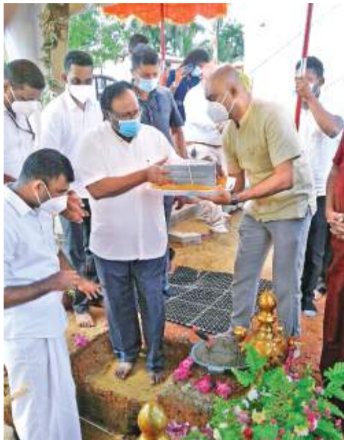
Public Security Minister Rear Admiral Dr. Sarath Weerasekera laying the foundation stone.
