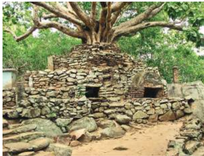
Bo-tree with massive stone wall
