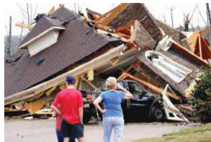
Residents survey the damage to homes after a tornado hit the town of Birmingham in Alabama, damaging a number of homes on Thursday.
