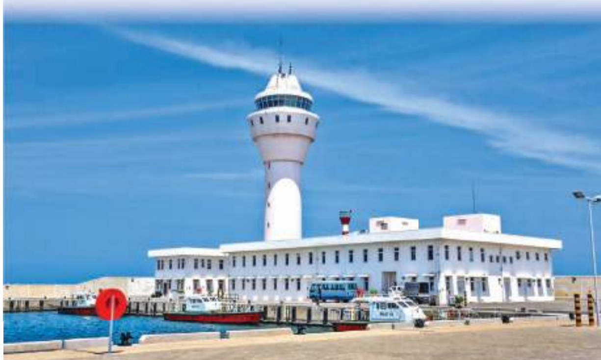
The newly constructed control tower, of the Colombo port. The Colombo port expansion is an ADB-supported project that helps raise the main port to international levels thus assisting small and large scale importers and exporters in their activities.
