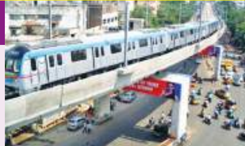
The Hyderabad metro rail.
