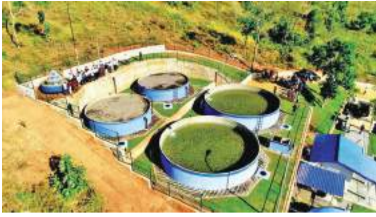
The Thalakolawewa Rural Water Supply Project.
