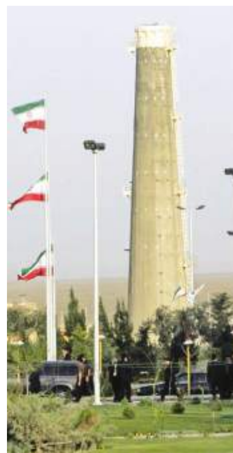
The Natanz Fuel Enrichment Plant in Iran.
