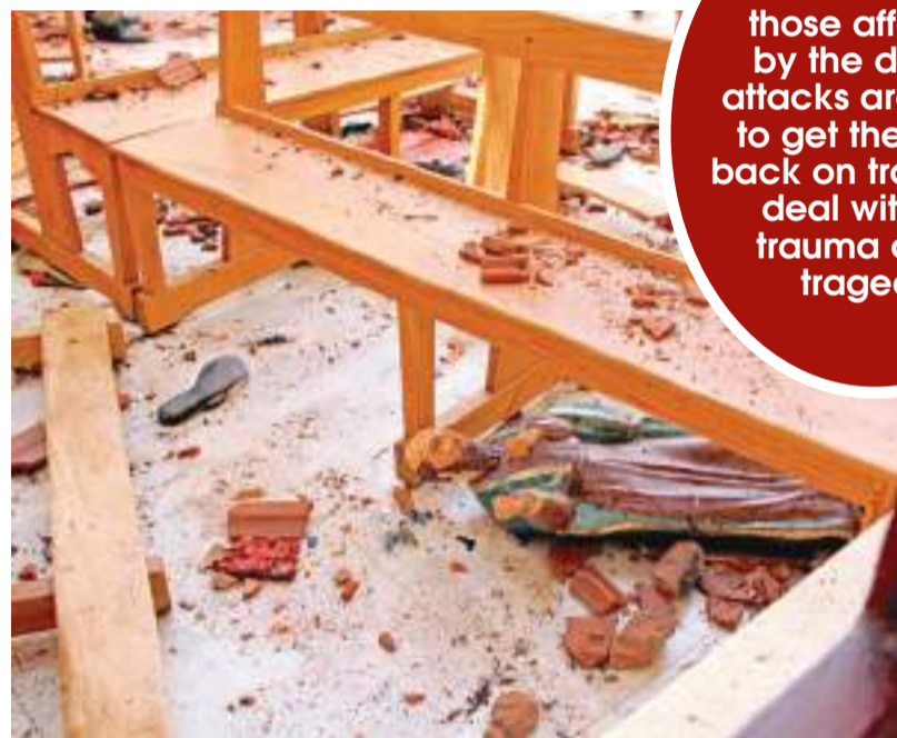
St. Sebastian's Church, Katuwapitiya after the blast.
