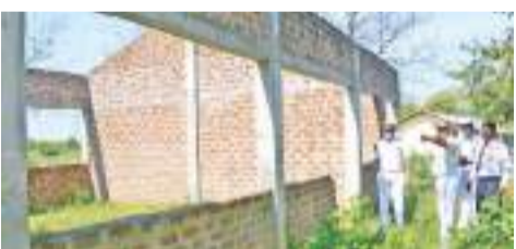
Navy personnel inspecting one of the underprivileged schools that is to be reconstructed.
