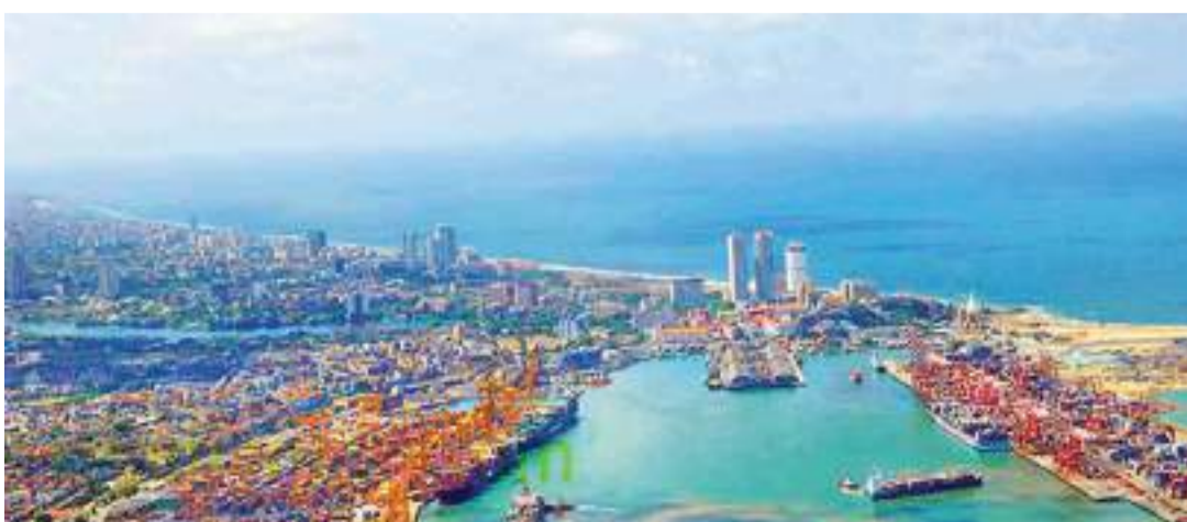
India is helping to develop the Western Container Terminal at the Colombo Port.
