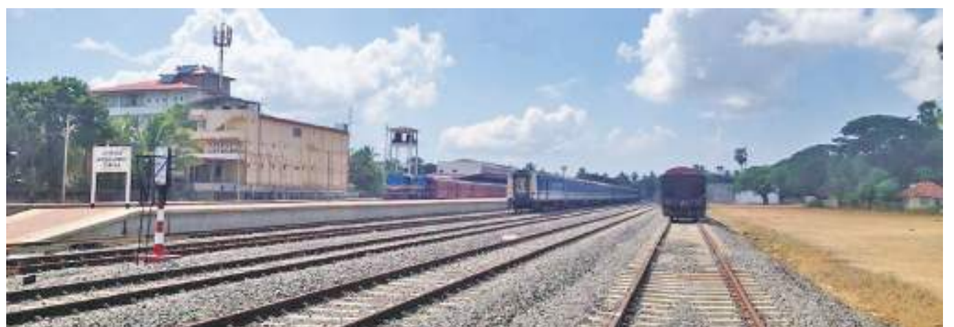
India assisted to renovate the Northern Railway Line in Sri Lanka.
