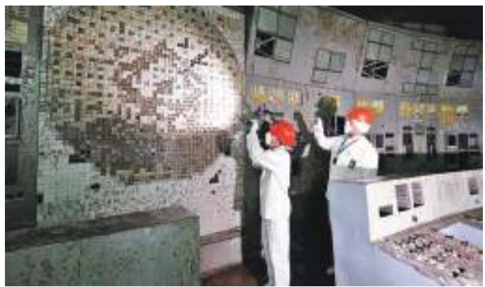
Inside the Chernobyl control room now
