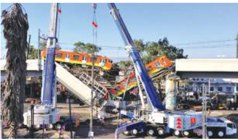
The damage caused after a railway overpass and train collapsed onto a road in Mexico City.
