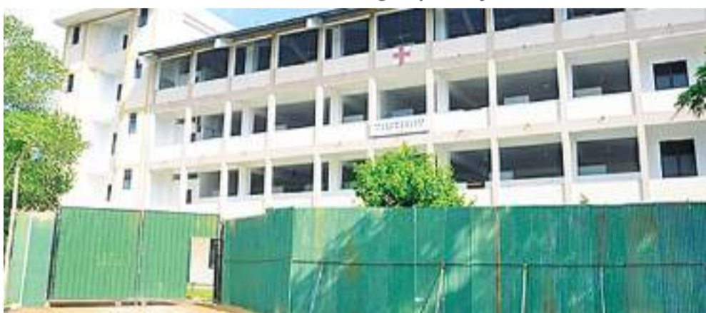
The four storied building which was converted into an Intermediate Care Centre for COVID-19 at the Boossa Naval Base
