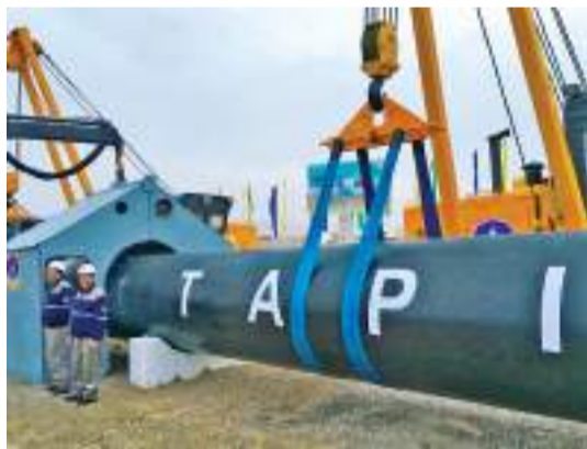
Construction work of the TAPI project on the Afghan section.
