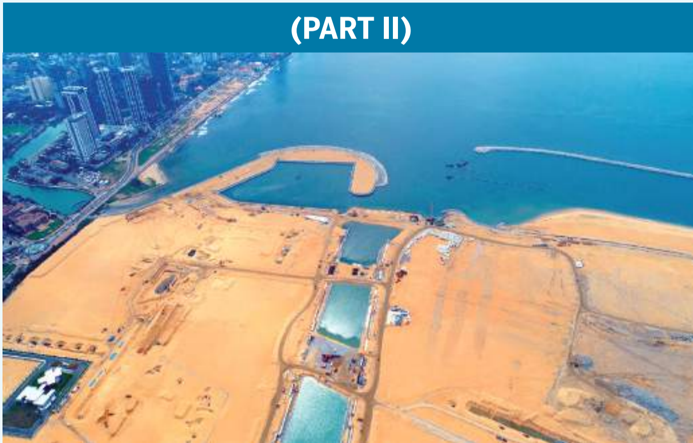
Port City under construction
