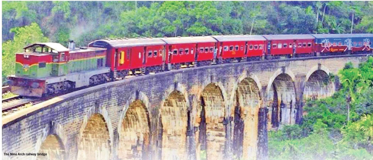
The Nine Arch railway bridge
