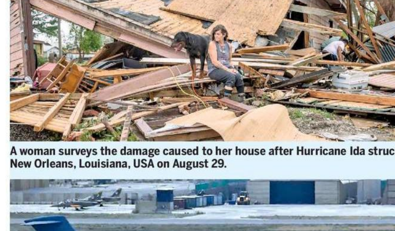
A woman surveys the damage caused to her house after Hurricane Ida struck New Orleans, Louisiana, USA on August 29.
