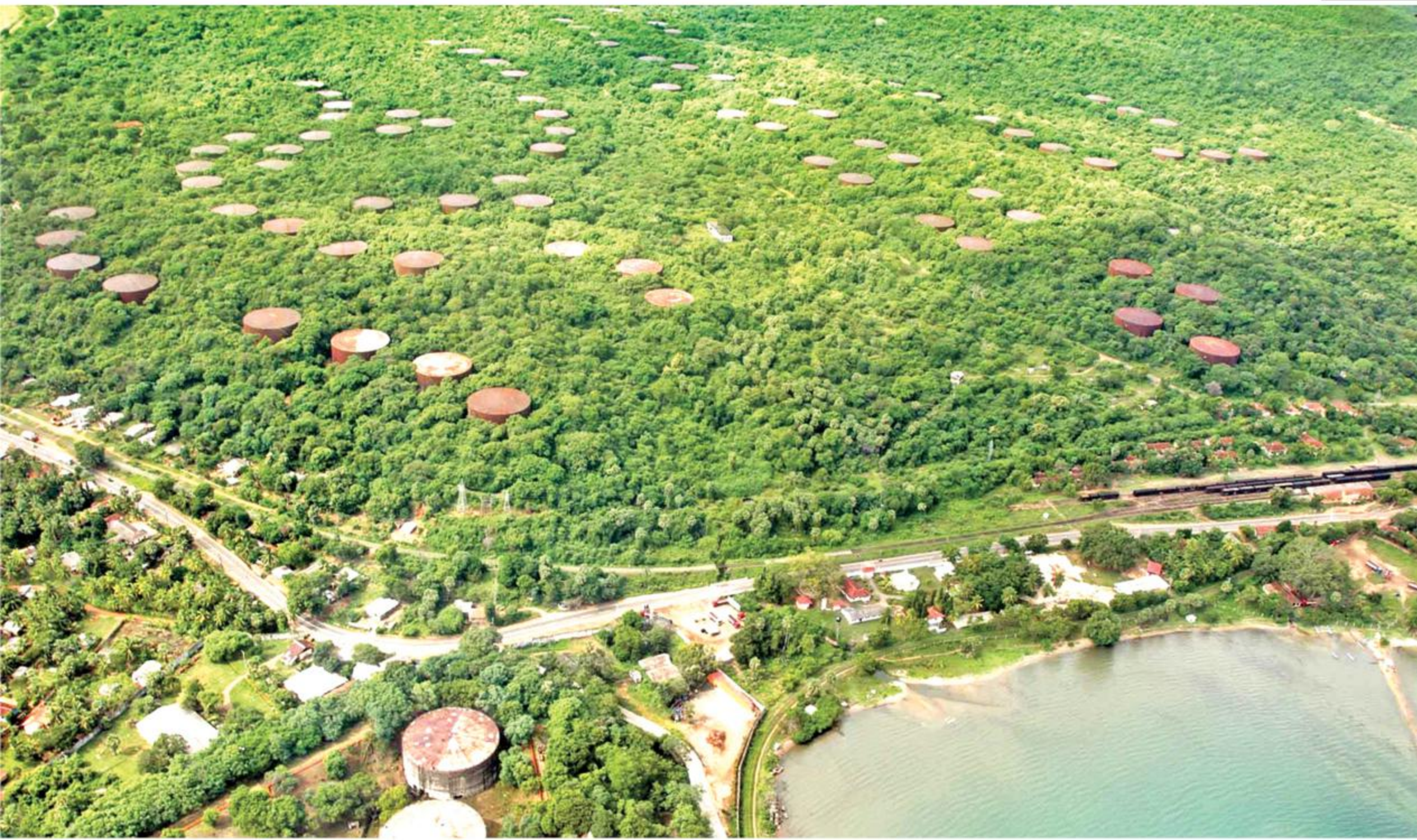
An aerial view of the China Bay Oil Tank Farm.
