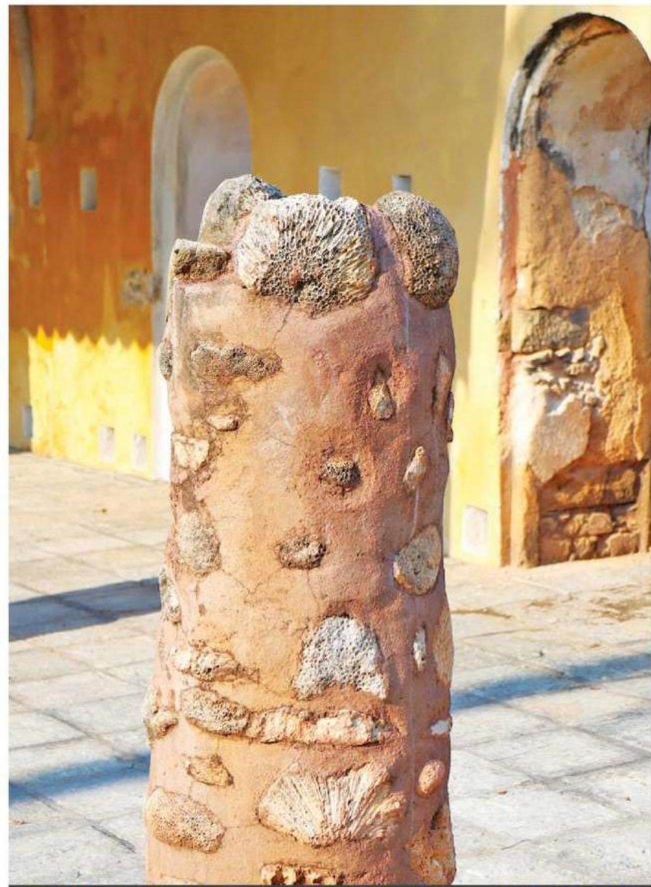
Coral in the columns came from the boat ballast as seen in The Black Fort
