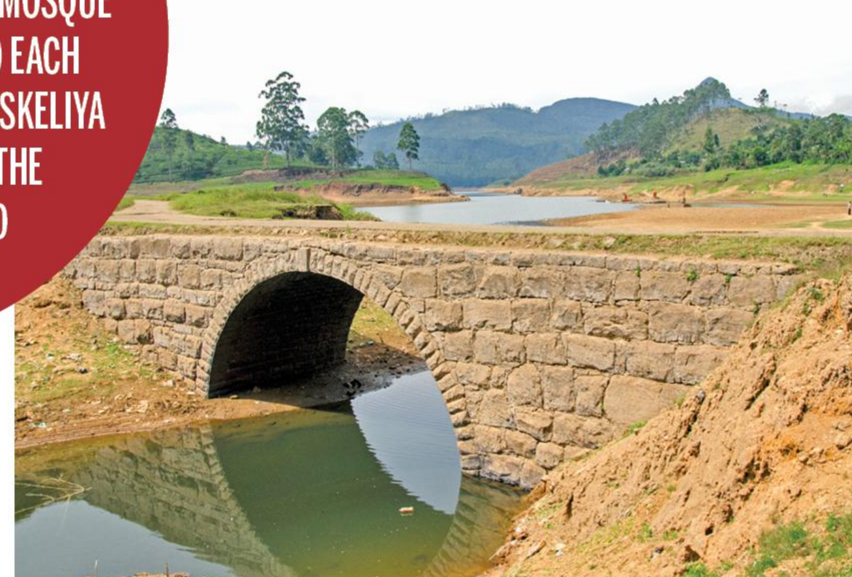
The British built arched stone bridge
