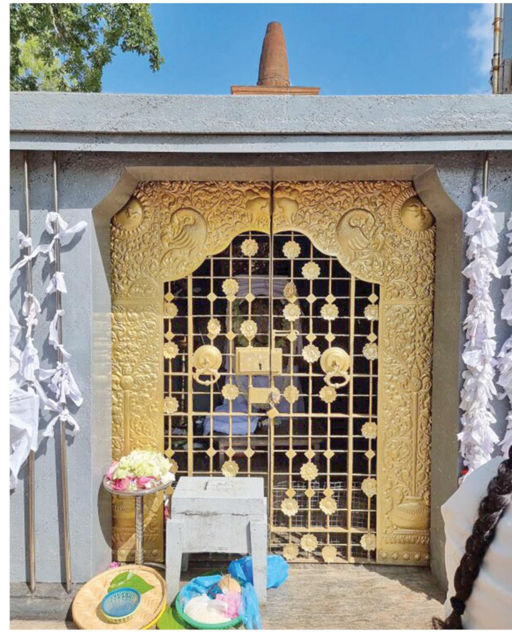
Worshippers' access to a Buddha statue in Anuradhapura is blocked by a gate for fear of damage or theft.
