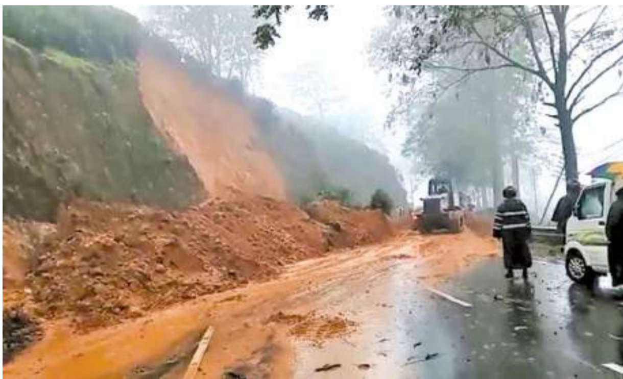
Traffic movement on the Hatton-Nuwara Eliya road came to a standstill for two hours when a huge mound of earth collapsed on the road in Nanuoya yesterday morning. Picture by Ranjith Rajapaksa, Hatton Corr.
