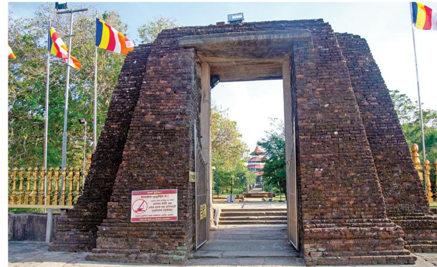
One of its ancient brick doorway
