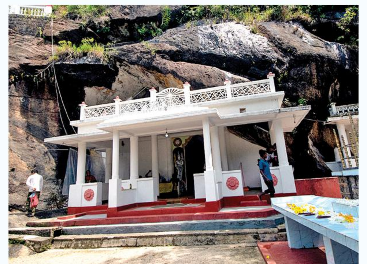
The front view of the entrance to the rock cave shrine
