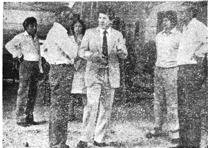
On his visit, the High Commissioner was taken round the Building site of the National Library. Also in the picture are, the Chairman, SLNLSB with other officials of the Board.
