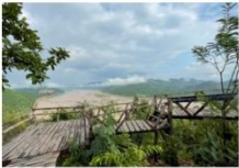
Pu Nong Peak facility
